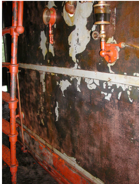
Allis Floor 3 North detail B, west side after treatment.
