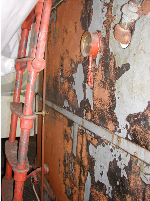
Allis Floor 3 North detail A, west side looking north before treatment.
