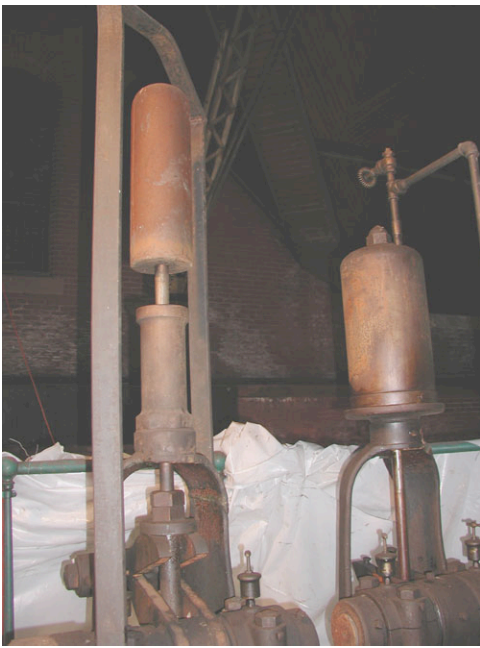
Allis Floor 4 North detail B before treatment.
