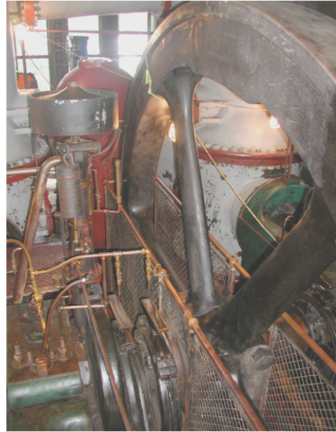
Worthington Floor 1 mid detail B, after treatment.
