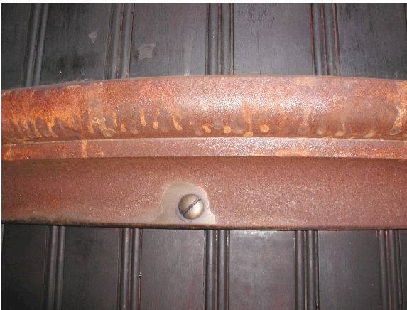
Figure C1. Originally plated surface, exhibiting extensive rust, Leavitt engine before treatment.
