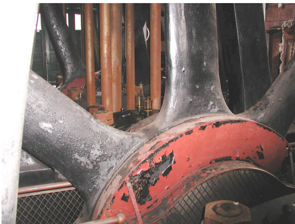
Figure G1. Paint failure at wheel of Allis engine before treatment.
