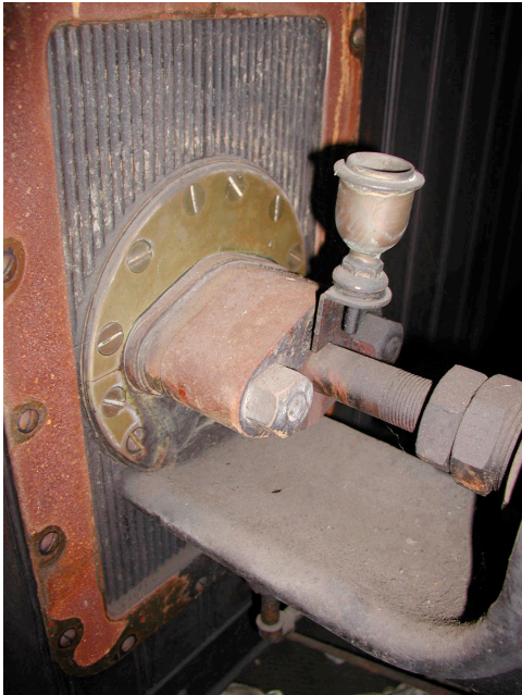
Figure D1. Galvanic corrosion (see surround plate) Leavitt engine before treatment.
