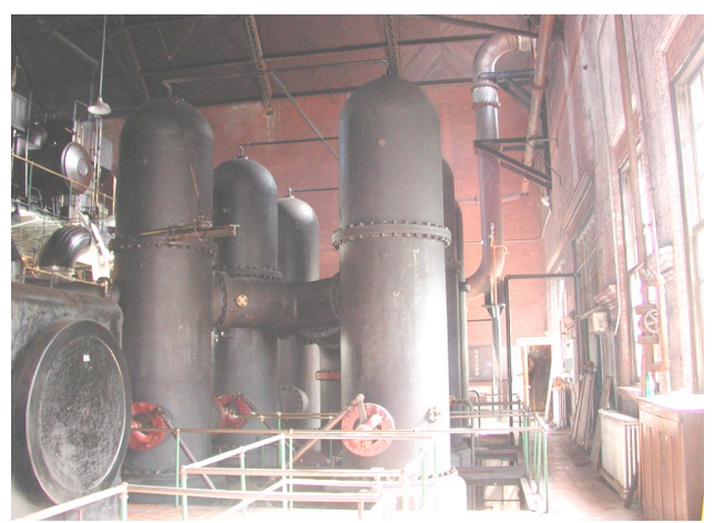
Leavitt engine (southwest) after treatment August 30, 2006.
