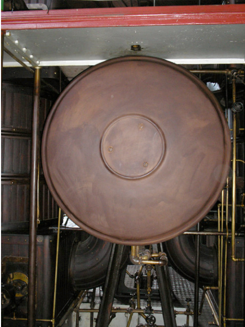
Figure H1. Leavitt engine rusted barrel end before CRC 3-36/microcrystalline wax treatment.
