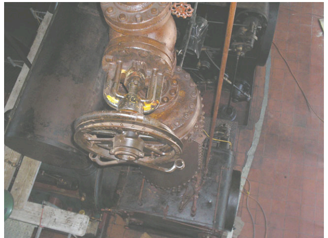
Worthington Floor 3 South detail D, after treatment.
