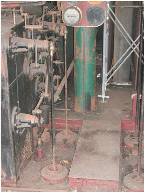
Worthington Floor 1 North detail C, looking north before treatment.
