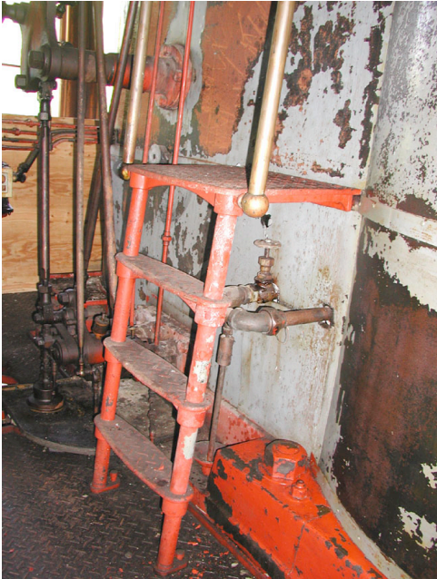
Allis Floor 3 South detail C, east side looking south before treatment.
