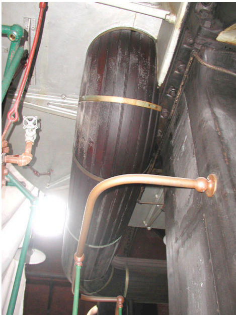
Leavitt Floor 2 North end detail G, east side before treatment.
