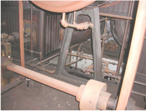
Leavitt Floor 3 North detail A, north side before treatment.
