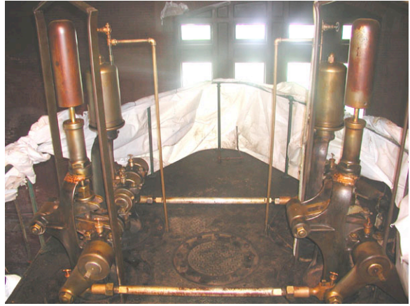
Allis Floor 4 North detail A after treatment.
