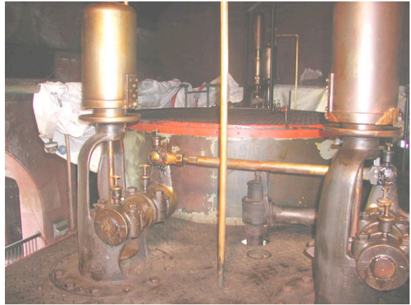
Allis Floor 4 mid detail C looking north after treatment.
