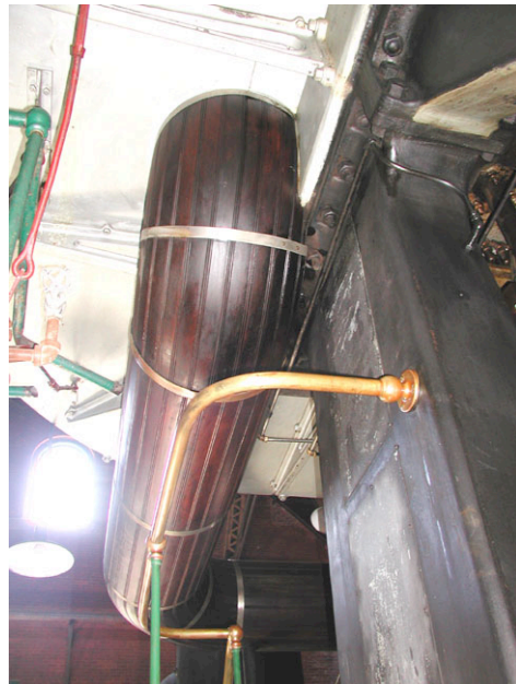
Leavitt Floor 2 North end detail H, after treatment.
