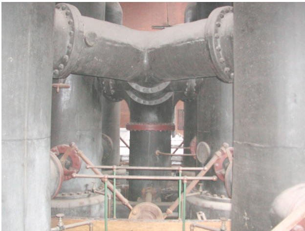
Leavitt Floor 3 South detail G, looking east before treatment.
