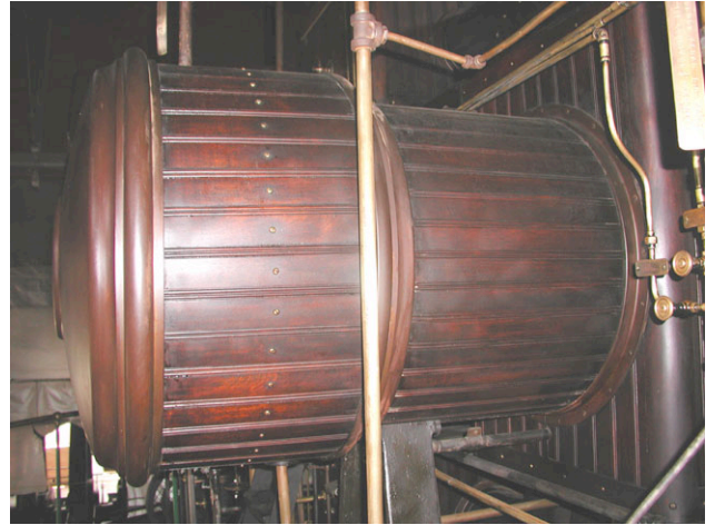
Leavitt Floor 3 North end detail F, south side after treatment.
