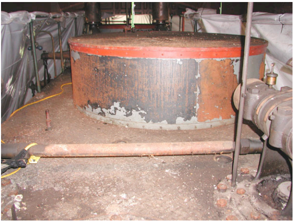
Allis Floor 4 North detail D barrel looking south before treatment.
