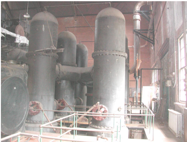
Leavitt engine (southwest) before treatment June 28, 2006.
