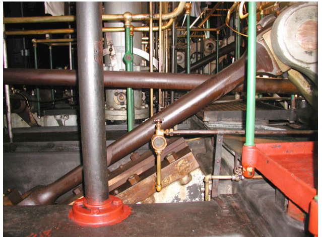
Leavitt Floor 2 North end detail D, east side after treatment.
