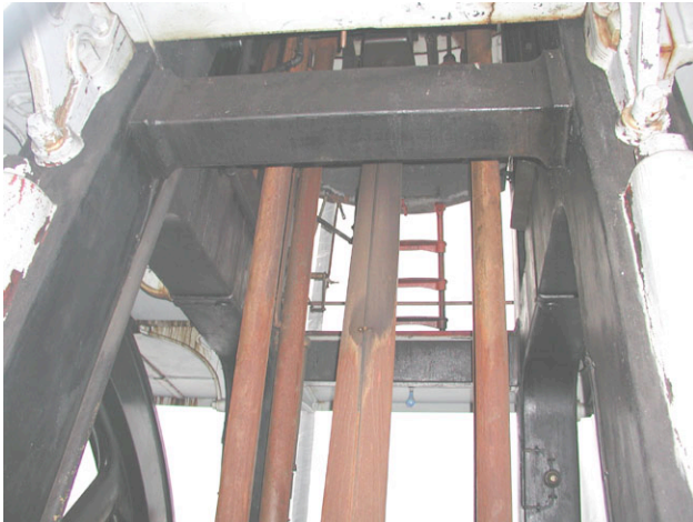
Allis Floor 1 North detail E, east side before treatment.
