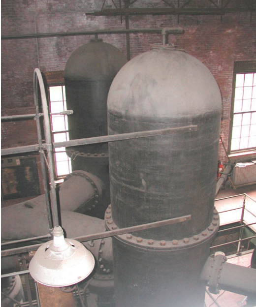
Leavitt Floor 4 South detail E, looking south before treatment.
