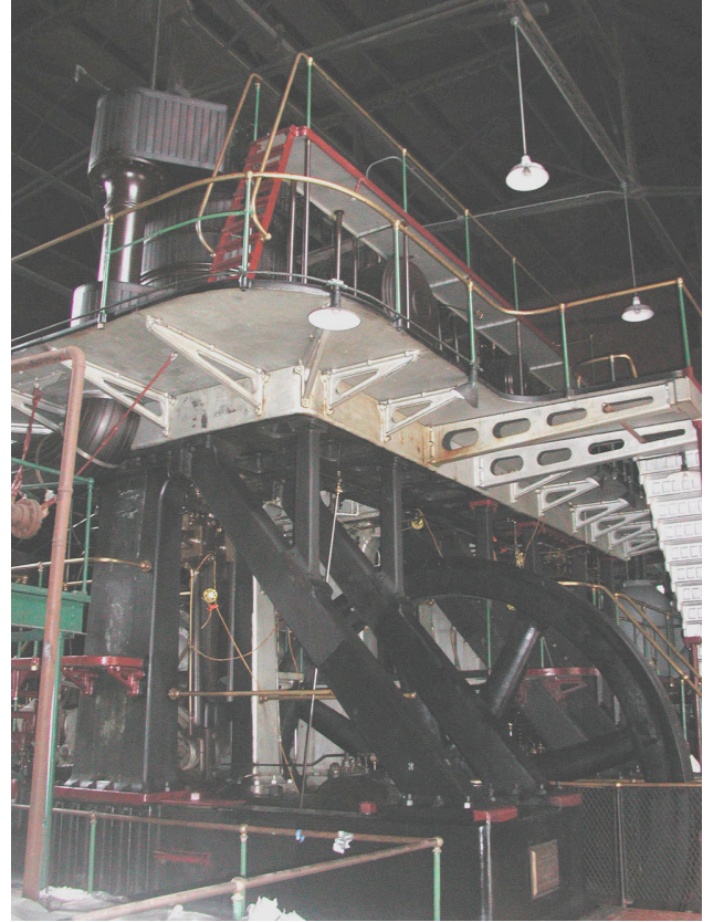
Leavitt engine (northeast) after treatment August 30, 2006.
