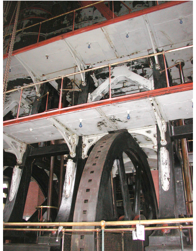
Allis engine (west) after treatment August 30, 2006.
