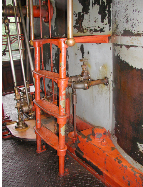
Allis Floor 3 South detail D, east side looking south after treatment.
