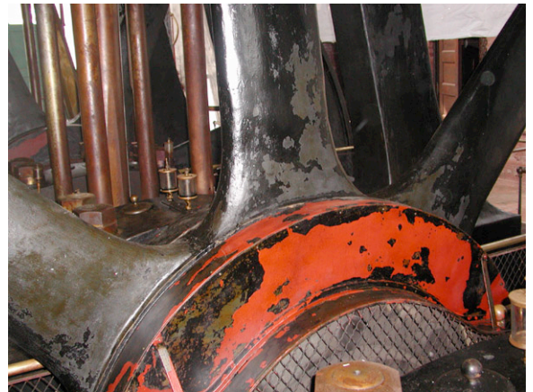
Figure G2. Paint failure at wheel of Allis engine after treatment.
