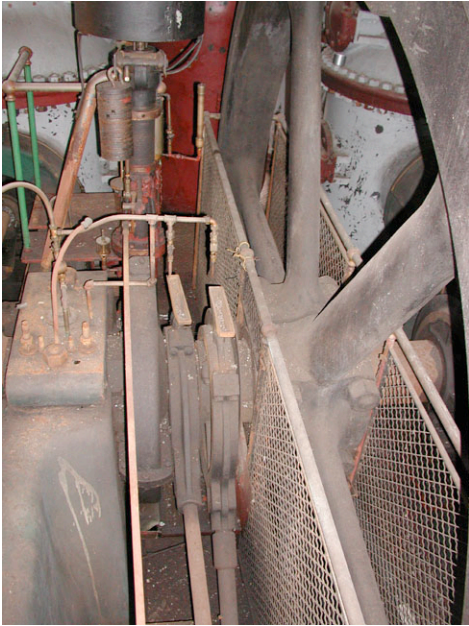
Worthington Floor 1 mid detail A, looking north before treatment.
