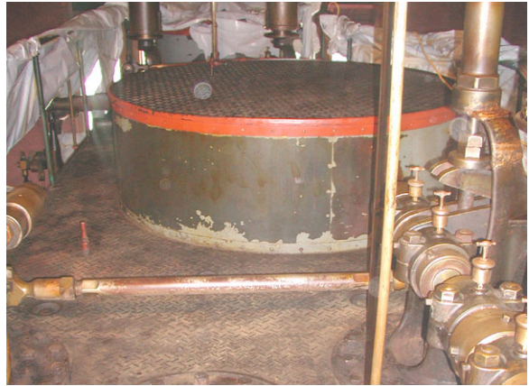
Allis Floor 4 North detail D barrel looking south after treatment.
