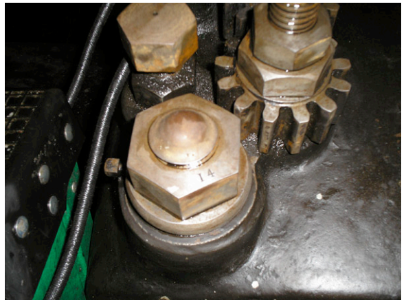
Figure I2. Leavitt engine, first floor bolt detail after cleaning. Note number now visible.
