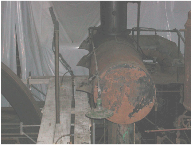
Worthington Floor 2 mid detail A, looking east before treatment.
