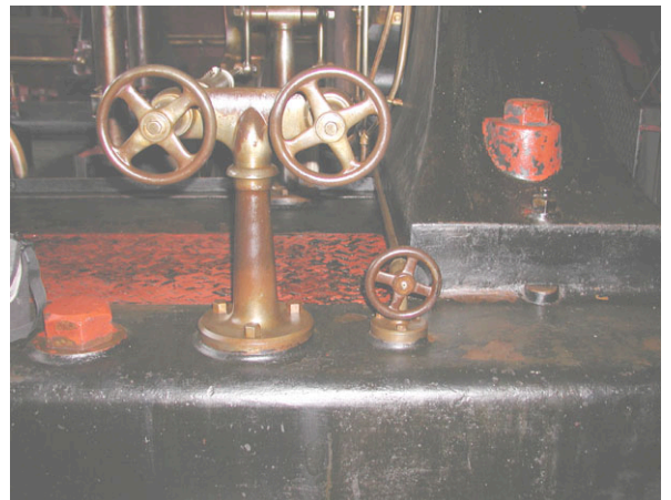
Allis Floor 1 South detail H, east side after treatment.
