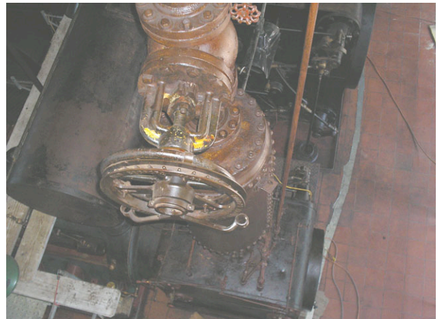
Worthington Floor 3 South detail D, after treatment.
