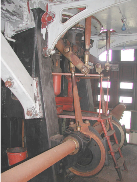
Allis Floor 2 South detail A, west side looking south before treatment.
